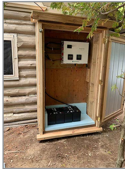
Power Pak and battery bank set up in a shed for some of our customers' cottage.
