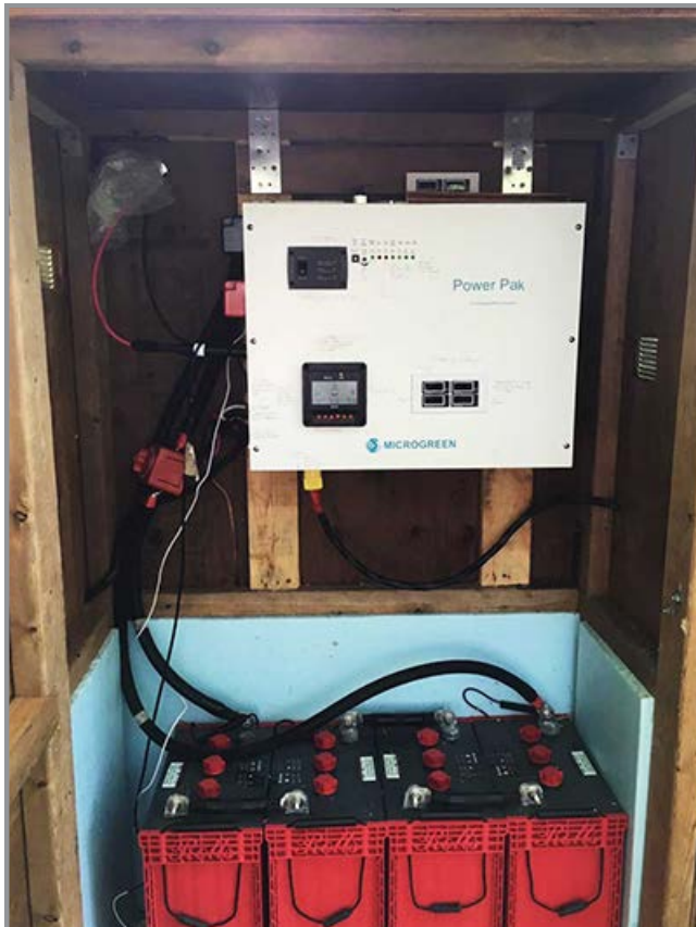
Power Pak and battery bank set up in a shed for some of our customers' cottage.
